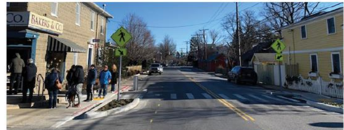
FIGURE 12. THIS RECENT INTERSECTION IMPROVEMENT ON CHESAPEAKE AVENUE SHORTENS THE CROSSING DISTANCE FOR PEDESTRIANS, CALMS VEHICULAR TRAFFIC, AND ADDS PLANTINGS.
