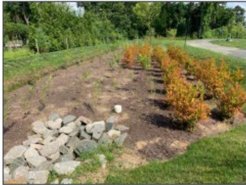
Bioretention facility SOURCE: CITY OF ALEXANDRIA
