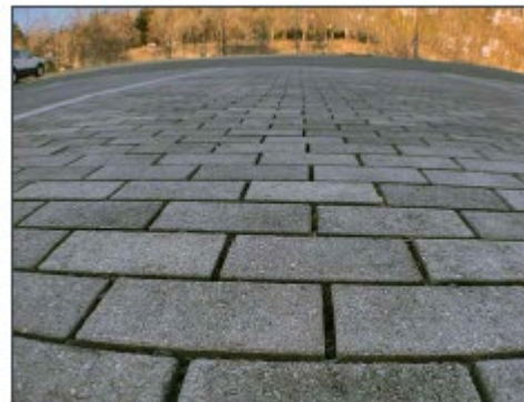
Permeable pavement SOURCE: CITY OF ALEXANDRIA
