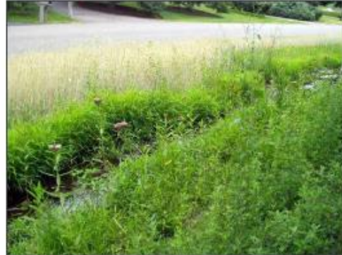
Wet swale SOURCE: CHESAPEAKESTORMWATER.NET
