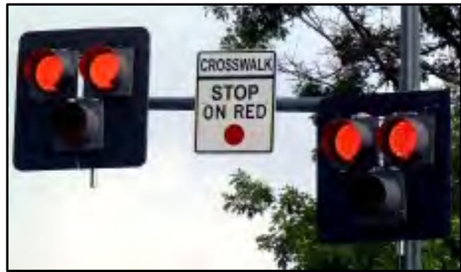
Figure 2.23: HAWK beacon at Georgia Avenue & Hemlock Street NW, Washington, D.C.
