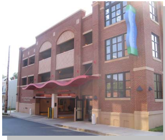
Knighton Parking Garage
