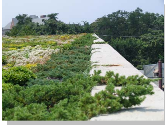
Green Roof on Severn Savings Bank Courtesy of: O'Doherty Group Landscape Architecture
