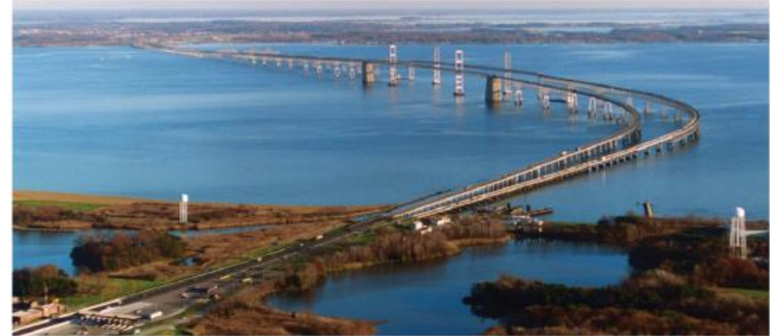
FIGURE 6-40: WITH OVER 60,000 DAILY TRIPS AND MANY MORE ON BUSY HOLIDAY WEEKENDS, THE BAY BRIDGE PROVIDES ENORMOUS ECONOMIC BENEFIT TO ANNAPOLIS AS WELL AS TRAFFIC CONGESTION. AS MDOT/SHA ADVANCES THE BRIDGE EXPANSION, ANNAPOLIS HAS A VESTED INTEREST IN DESIGNS THAT WILL IMPROVE TRAFFIC MANAGEMENT AND PROMOTE MORE ALTERNATIVE MODES OF CROSSING.
