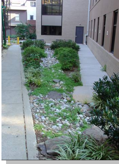
Rain garden at Hillman Parking Garage
