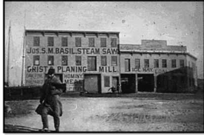
Archival Photo - Jos. Basil Steam Saw Grist and Planing Mill ca. 1895 at City Dock at foot of Main street. HA Scanned Image,
