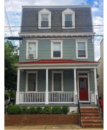
6 Units – Cathedral Street
