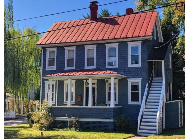
2 Units – Washington Street
