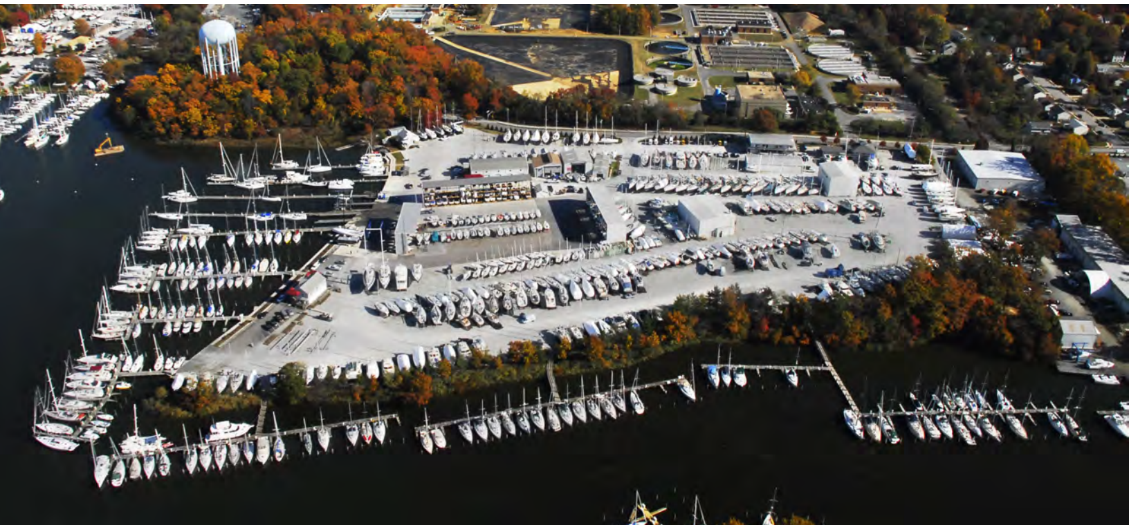
Boat lifts and boat storage at Bert Jabin Yach Yard in the WMI District
