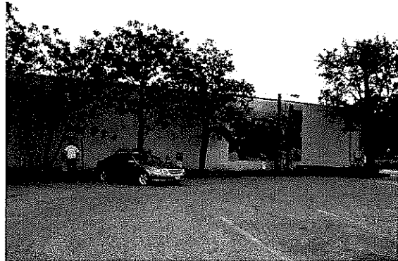
City Owned Parking Lot
