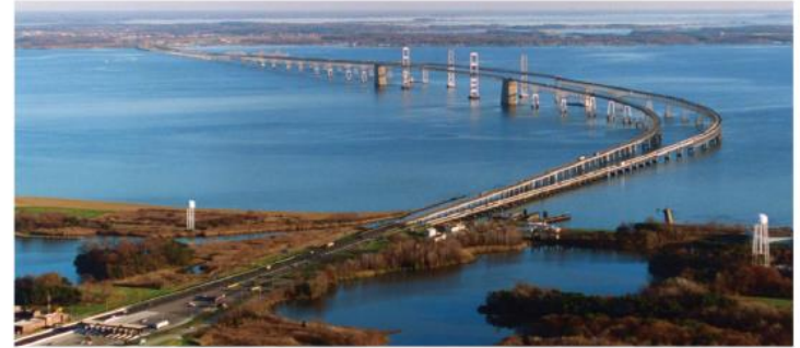
FIGURE 6-40: WITH OVER 60,000 DAILY TRIPS AND MANY MORE ON BUSY HOLIDAY WEEKENDS, THE BAY BRIDGE PROVIDES ENORMOUS ECONOMIC BENEFIT TO ANNAPOLIS AS WELL AS TRAFFIC CONGESTION. AS MDT/SHA ADVANCES THE DTHE BRIDGE EXPANSION, ANNAPOLIS HAS A VESTED INTEREST IN DESIGNS THAT WILL IMPROVE TRAFFIC MANAGEMENT AND PROMOTE MORE ALTERNATIVE MODES OF CROSSING.
