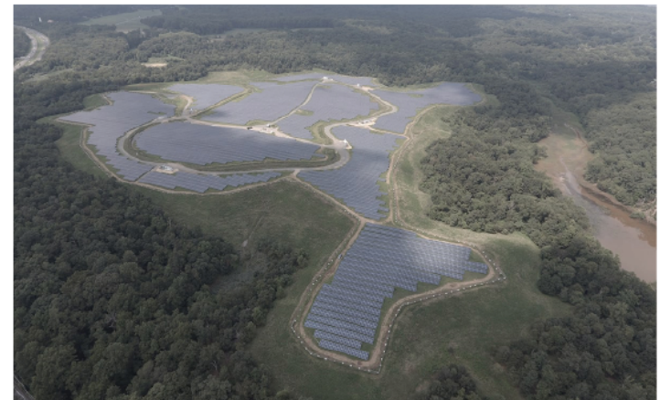
FIGURE 9-27: ACCORDING TO THE EPA, THE ANNAPOLIS SOLAR PARK AT WATERWORKS PARK IS THE LARGEST SOLAR INSTALLATION ON A CLOSED LANDFILL IN NORTH AMERICA.
