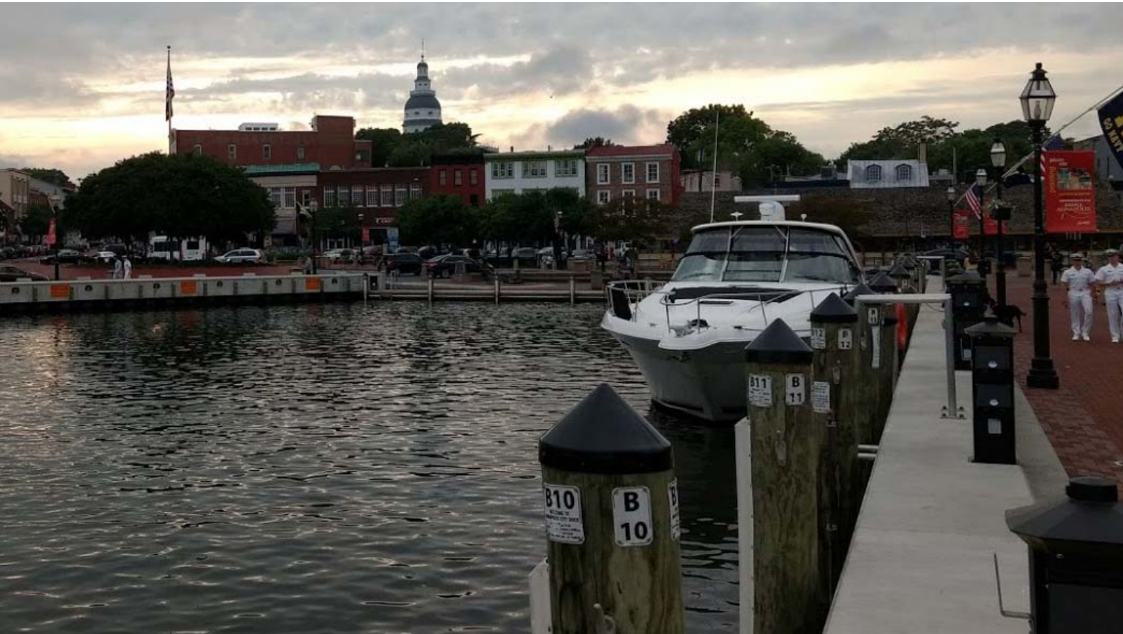
Annapolis City Dock Bulkhead, May, 2017
