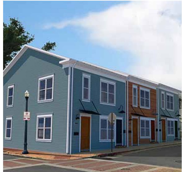
FIGURE 4-6: NEW AFFORDABLE HOUSING FOR VETERANS ON CLAY STREET
