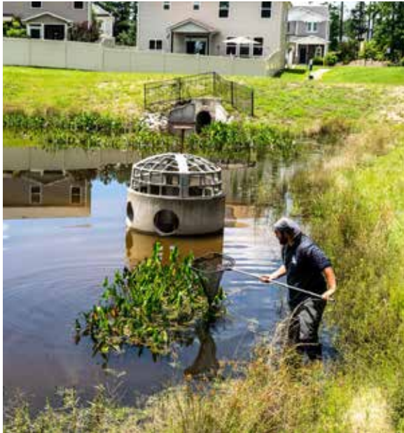
FIGURE 7-25: ROUTINE MAINTENANCE OF STORMWATER MANAGEMENT FEATURES IS CRITICAL TO ENSURING THAT THE FEATURES FUNCTION AS DESIGNED.
