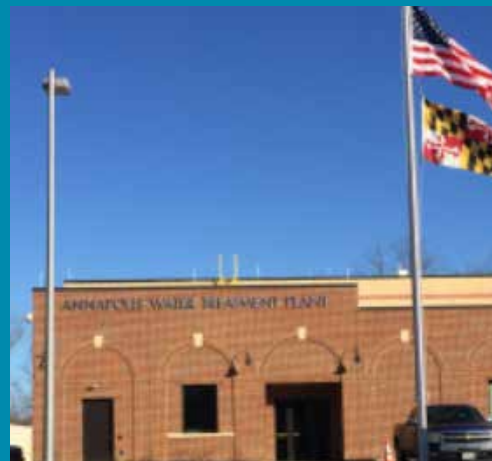
FIGURE 10-2: WATER TREATMENT PLANT
