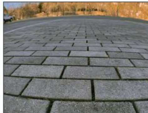
Permeable pavement SOURCE: CITY OF ALEXANDRIA
