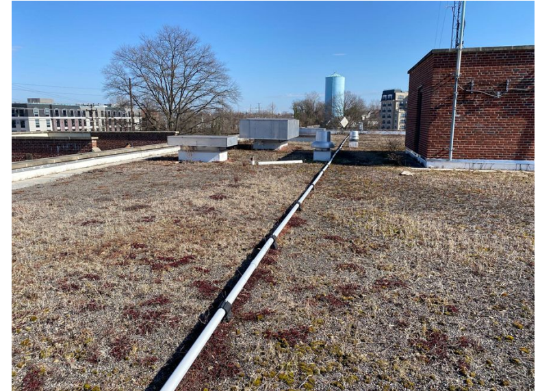
City Facilities - Green Roof Maintenance
