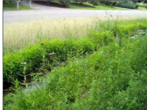
Wet swale SOURCE: CHESAPEAKESTORMWATER.NET
