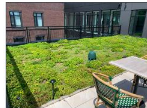
Vegetated green roof SOURCE: CITY OF ALEXANDRIA
