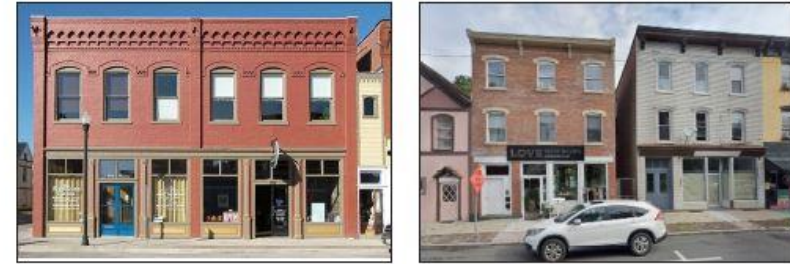
Figure 405.12.G: Examples of Live/Work Buildings:
