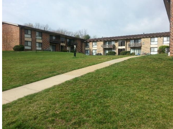
NSA_12 – Forest Hills Apartments
