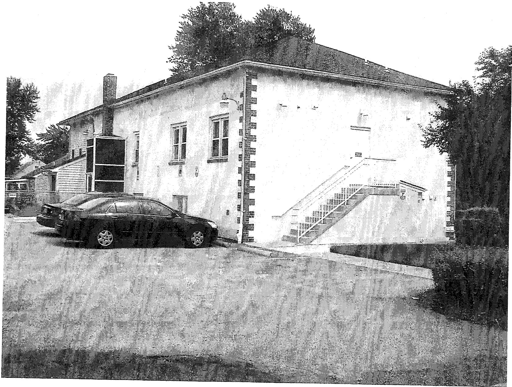
Community Health Center at Parole, Exterior View of West and North Elevations, Looking SE
