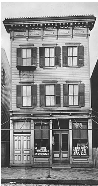
Figure 30. Italianate facade with bracketed cornice, 118 Main Street, 1888-95. During the second half of the nineteenth century, the vitality of commercial enterprise was expressed in the decoration of street facades. Bracketed cornices, door and window hoods, and elaborate storefronts embellished new and remodeled structures. (Mame Warren Collection, Maryland State Archives, MSA SC 985-112)
