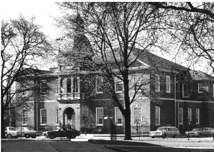
Figure 63. Anne Arundel County Courthouse, Church Circle. Despite its large size, the courthouse facade facing Church Circle has a human scale because of the skillfull changes in plane and additive massing.
