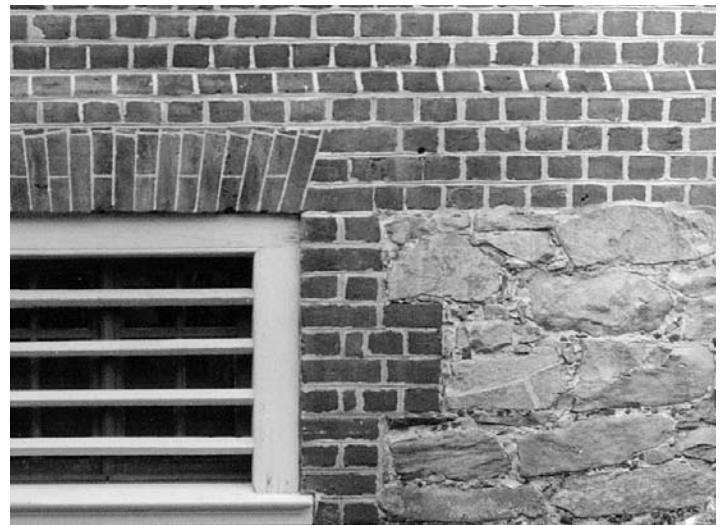
Figure 79. Detail of William Paca House foundation and cellar window. The all-header brick bond and the pebbles in the stonework mortar joints (galleting) are distinctive Annapolis details which require skilled craftsmanship to preserve.
