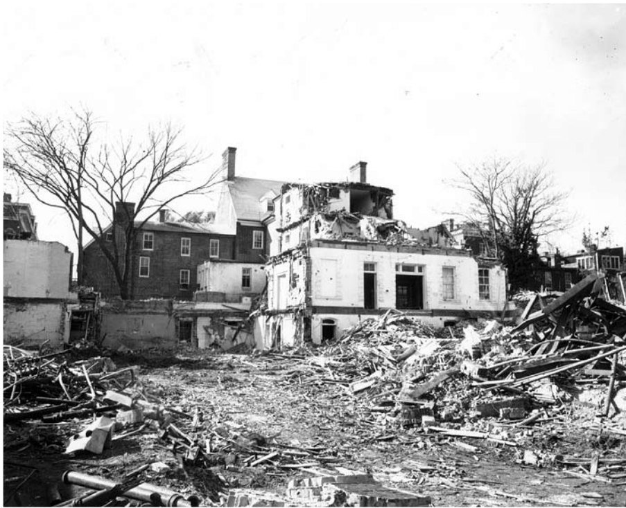
Figure 3. William Paca House, 186 Prince George Street (1763-1765). Left: View from northeast during demolition of Carvel Hall Hotel. Below: Restored garden and facade. (Marion Warren Collection, Maryland State Archives. Left: MSA 1890-2021-3; below: MSA SC 1890-3526 [detail].)
