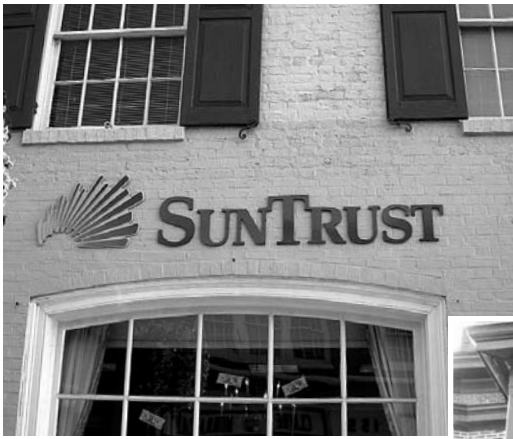
Above: example of free standing, raised lettering applied directly to the wall.
