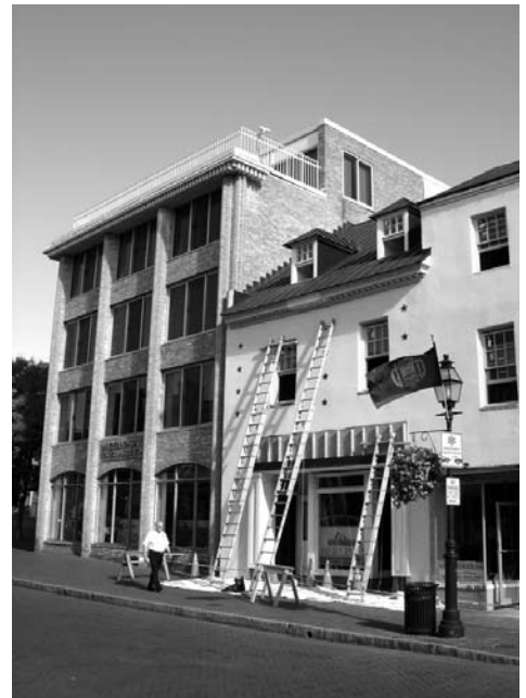
Figure 64 Example of inappropriate infill. The building on the left is not integrated with the buildings that surround it. (Photograph courtesy of Donna C. Hole)
