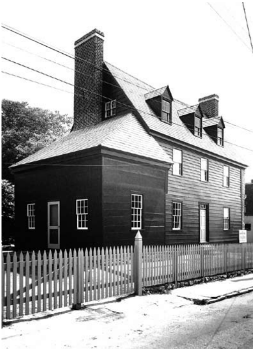
Figure 20b. Shiplap House, 18 Pinkney Street, c. 1715. The steep roof, mix of three types of siding, small windows, and single pile floor plan are characteristic of early eighteenth century vernacular dwellings in Annapolis. (Marion Warren Collection, Maryland State Archives, MSA SC 1890-243)
