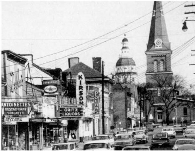
Figure 5. West Street Comparative views, 1965 and 1977. The Annapolis Urban Renewal Authority repaved West Street, planted street trees, and buried utility lines. Following this public initiative, many building owners restored and reconstructed their building exteriors. (Marion Warren Collection, Maryland State Archives. Left: MSA SC 1890-1693; below: MSA SC 1890-3448.)
