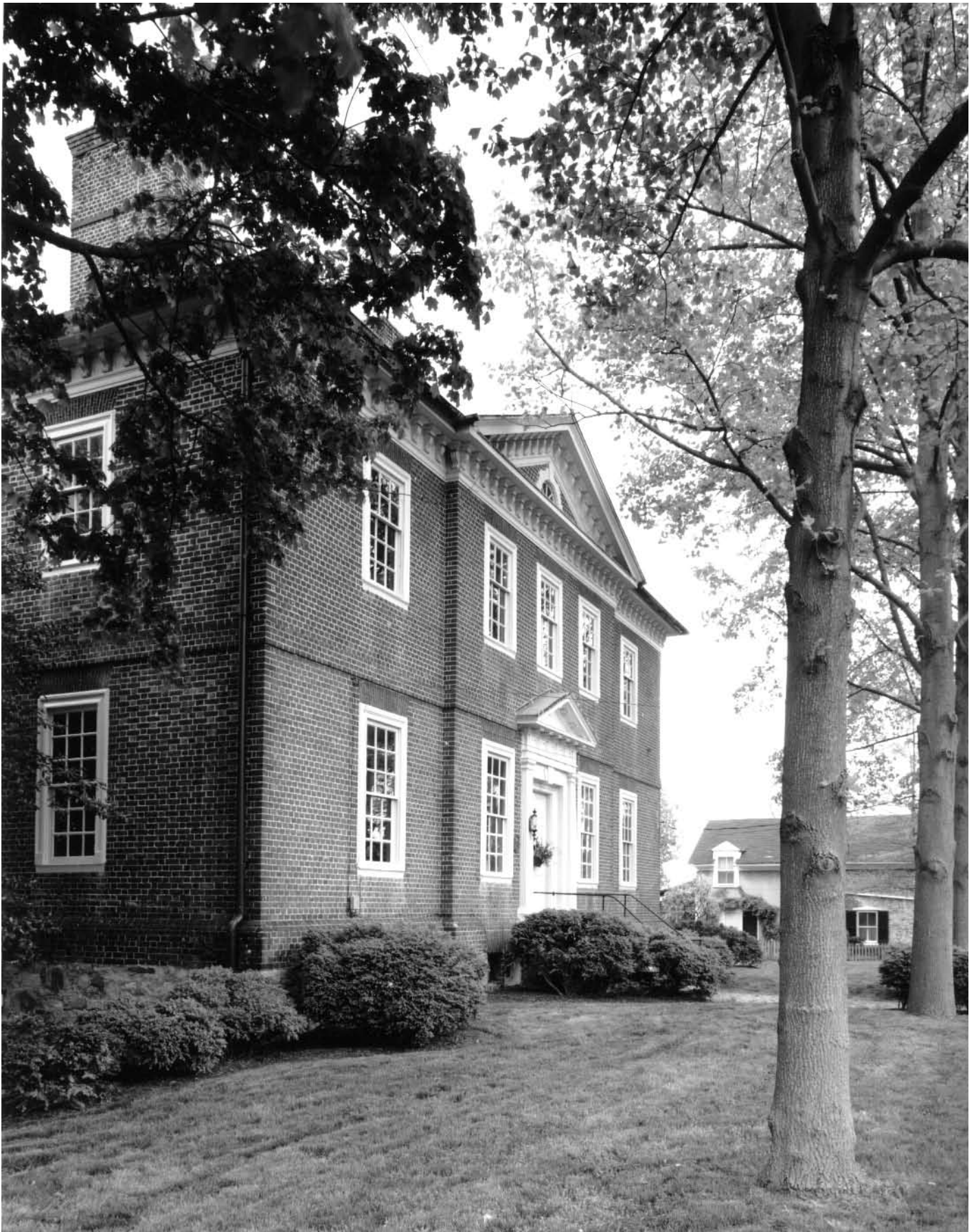
Figure 37. Upton Scott House, 4 Shipwright Street, 1762-63. The Upton Scott House was described as “the best town house in America” by Daniel Dulany shortly after its completion. (Willie Graham, Colonial Williamsburg Foundation, 1996)
