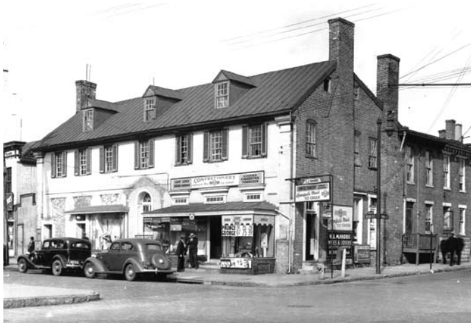
Figure 73. Historical photographs such as this view of Middleton Tavern, 2 Market Space, provide invaluable information regarding the earlier appearance of historic buildings. (Courtesy of Historic American Buildings Survey, Library of Congress. E. Pickering, 1936)
