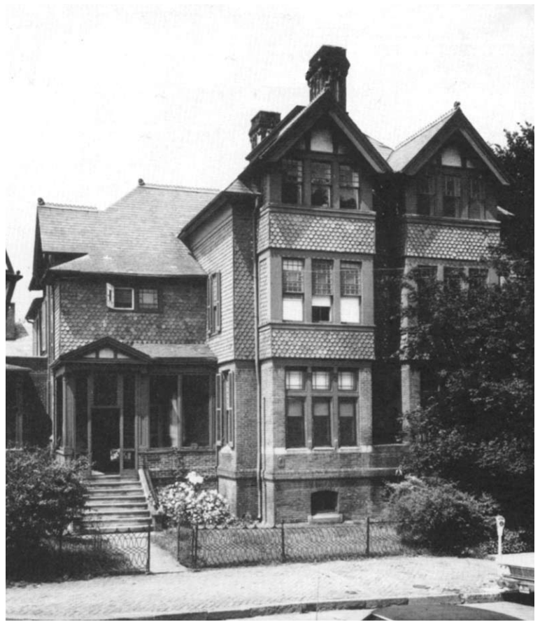
Figure 50. 86-88 State Circle, 1878. This pair of semi-detached dwellings skillfully employs the Queen Anne Revival use of projecting bays, paneled brick chimneys, specialized window shapes, and picturesque composition. (Marion Warren Collection, Maryland State Archives, MSA SC 1890-2897)
