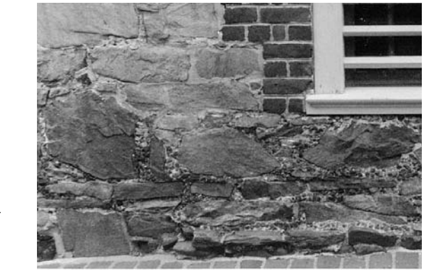
Figure 18 (above). Detail of galleting, William Paca House.
