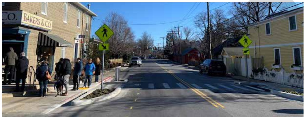
FIGURE 6-16: THIS RECENT INTERSECTION IMPROVEMENT ON CHESAPEAKE AVENUE SHORTENS THE CROSSING DISTANCE FOR PEDESTRIANS, CALMS VEHICULAR TRAFFIC, AND ADDS PLANTINGS.
