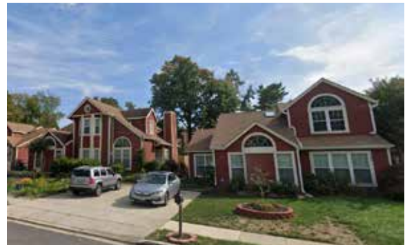
FIGURE 5-5: SINGLE FAMILY DETACHED HOMES NEAR EDGEWOOD ROAD
