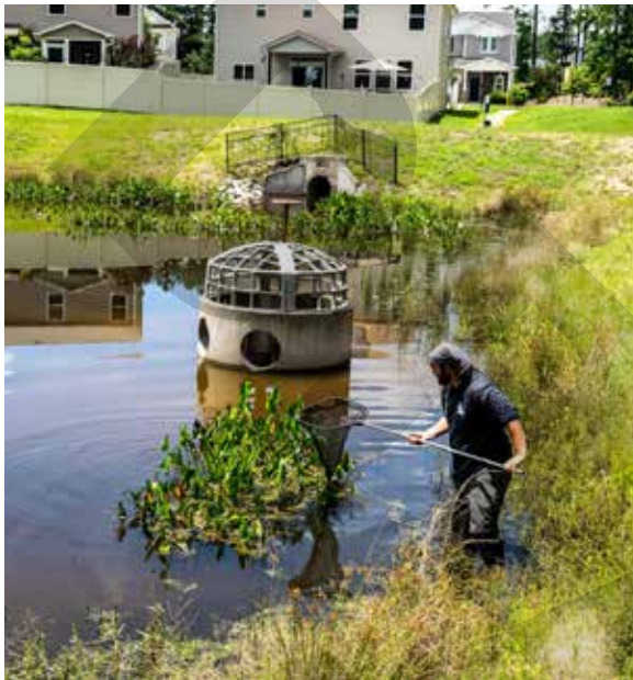
FIGURE 7-25: ROUTINE MAINTENANCE OF STORMWATER MANAGEMENT FEATURES IS CRITICAL TO ENSURING THAT THE FEATURES FUNCTION AS DESIGNED.
