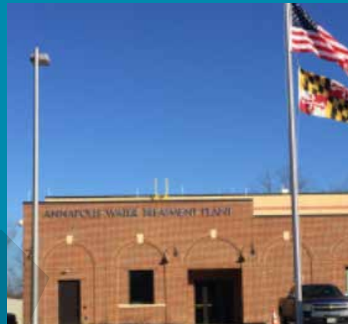
FIGURE 10-2: WATER TREATMENT PLANT
