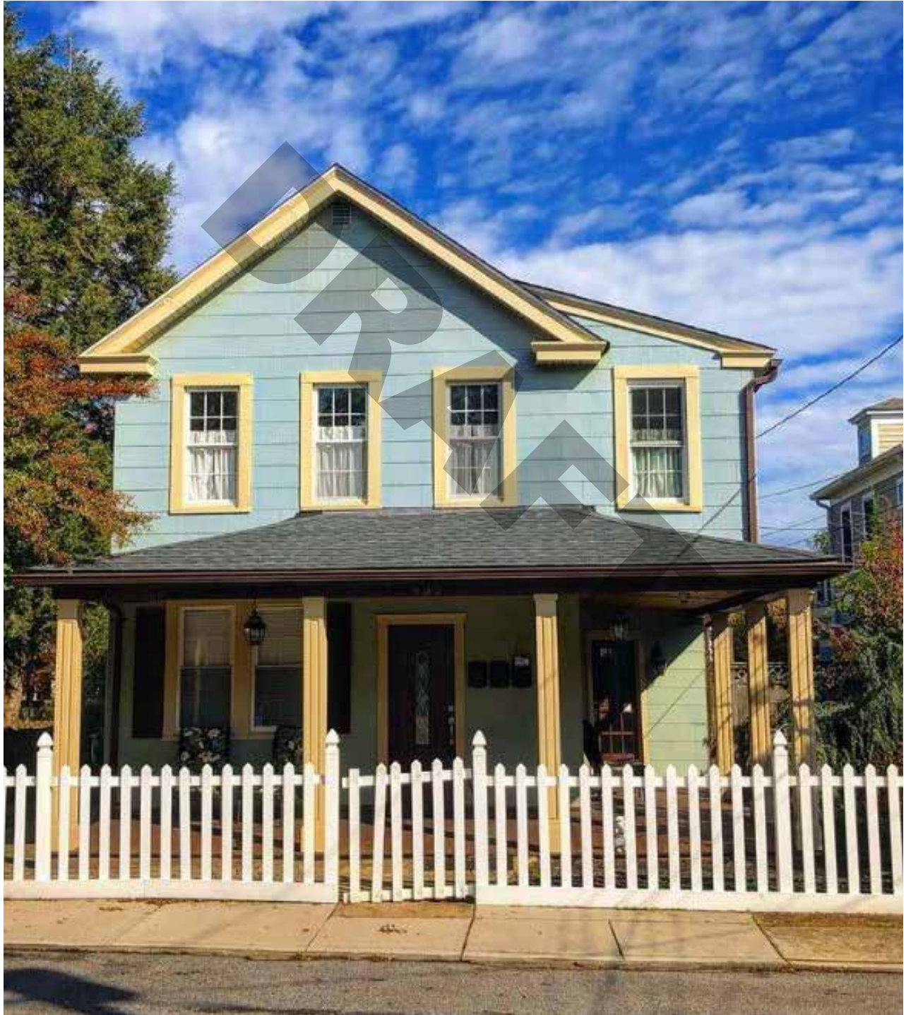
FIGURE EX-45: THIS HOUSE IN EASTPORT COULD BE MISTAKEN FOR A SINGLE FAMILY HOME BUT IN FACT CONTAINS THREE APARTMENTS AND IS IN KEEPING WITH THE NEIGHBORHOOD CHARACTER.
