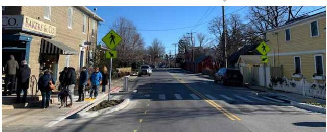
FIGURE 6-15: THIS RECENT INTERSECTION IMPROVEMENT ON CHESAPEAKE AVENUE SHORTENS THE CROSSING DISTANCE FOR PEDESTRIANS, CALMS VEHICULAR TRAFFIC, AND ADDS PLANTINGS.
