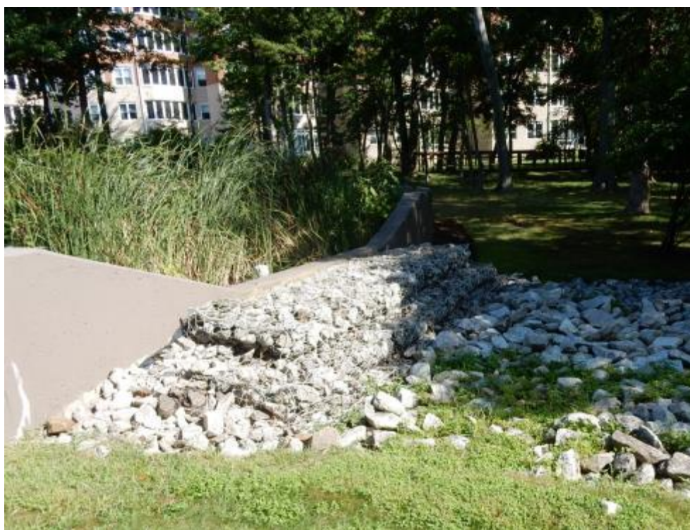
Existing Pond at BayWoods of Annapolis Overflow Weir and Outfall Protection (facing northwest)
