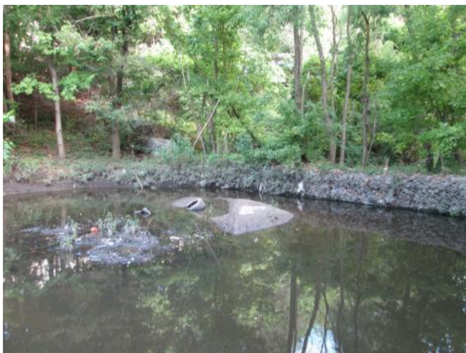
Existing Wet Pond Gabion Outlet Structure
