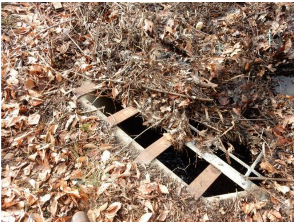
Existing Ambridge Pond Principal Spillway (with 36-inch pipe through embankment)
